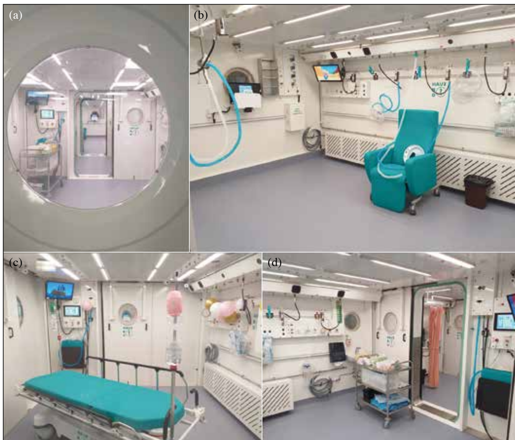
Figure 1. (a) An overview of the three locks of the hyperbaric oxygen chamber. (b) The chamber for ambulatory patients with central retinal artery occlusion who sit on the sofa and wear a transparent hood that delivers oxygen during treatment. (c) A stretcher is placed in the intensive care unit lock. Balloons are used to demonstrate pressurization and depressurization. (d) A toilet is located behind the orange curtain. Patients are kept under pressurisation while going to toilet.
