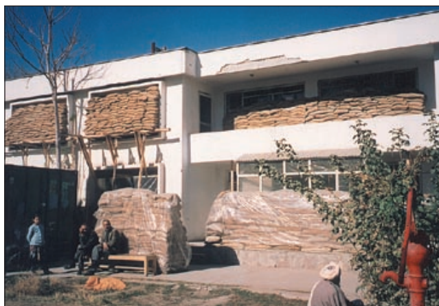
Figure 5. One of the present NOOR Eye Hospitals, packed with sandbags for protection.
